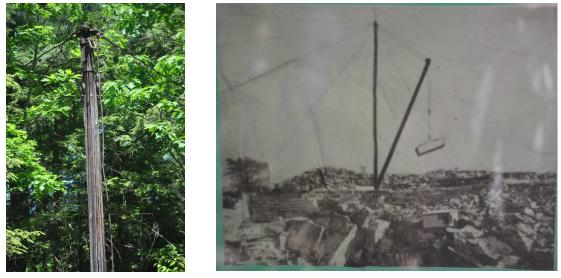
The remains of the derrick (left) used to lift the cut granite and what it looked like in operation (above) with the boom (no longer present) attached.
